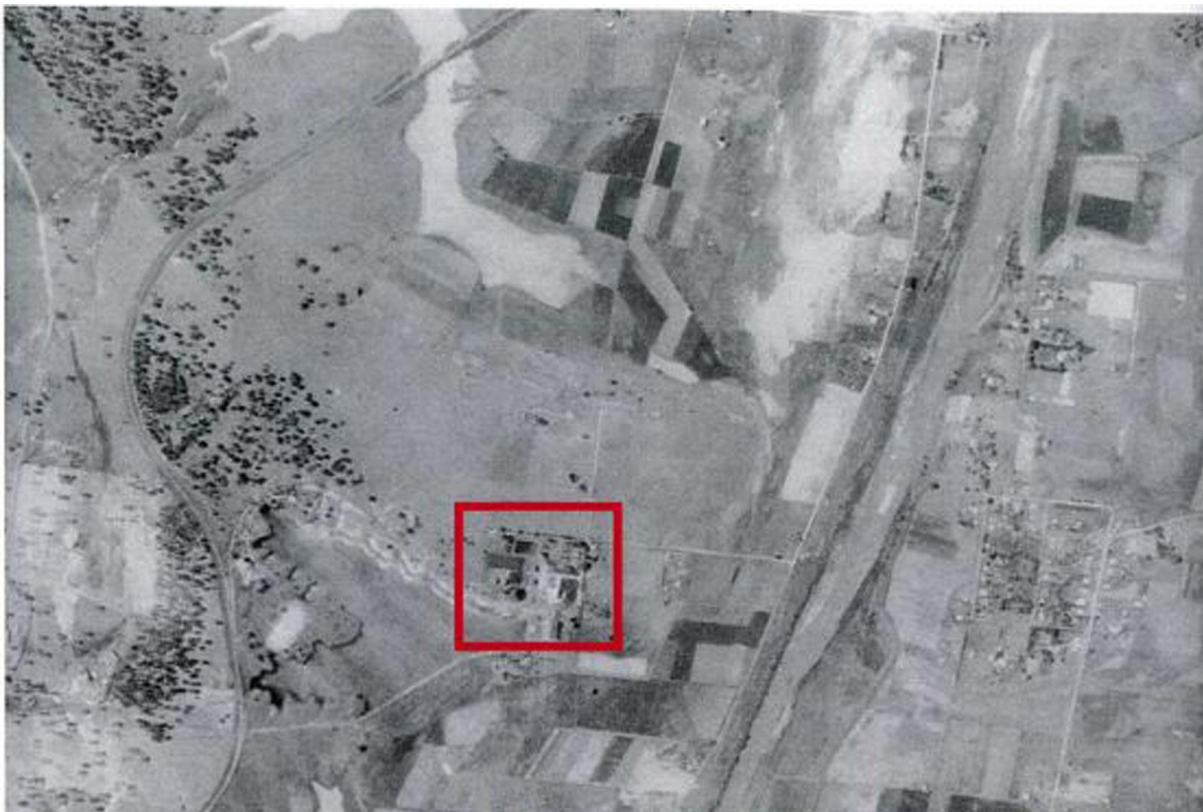
1958 aerial photo of the power station, the siding can be seen looping to the left.
