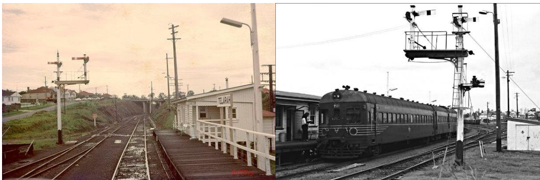
Two uncredited shots of the original station, probably taken in the 1980s
